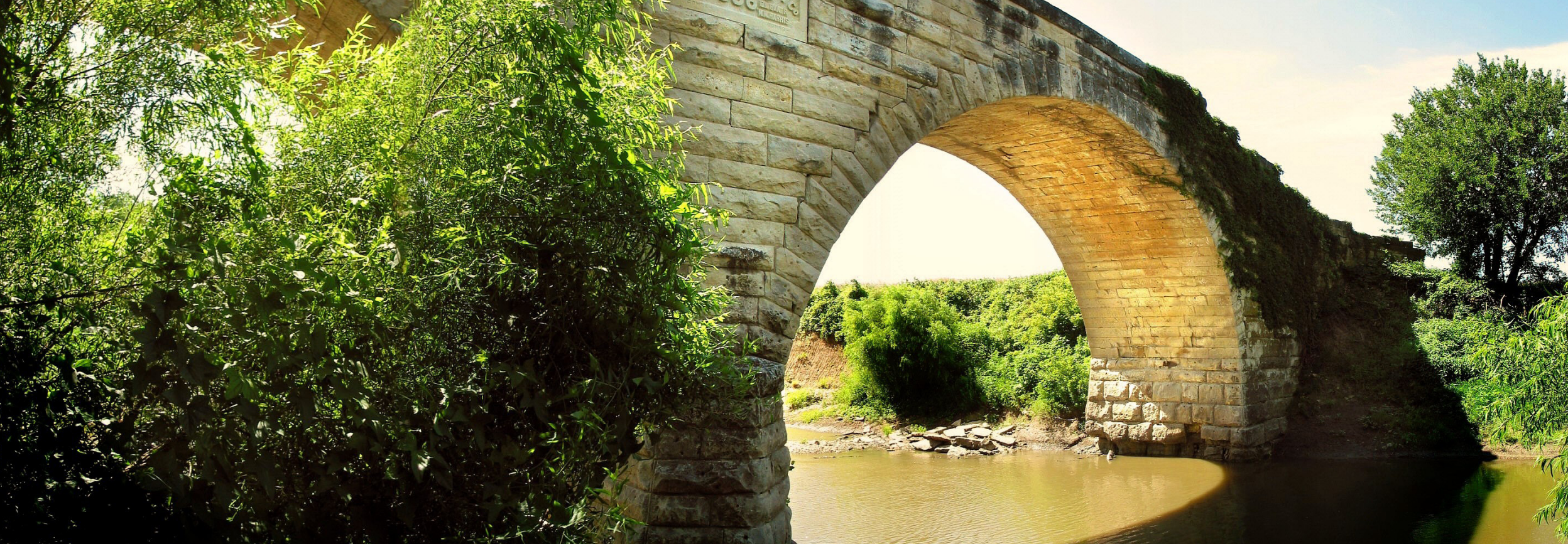
CLEMENTS BRIDGE — LOW WATER Dave Leiker
