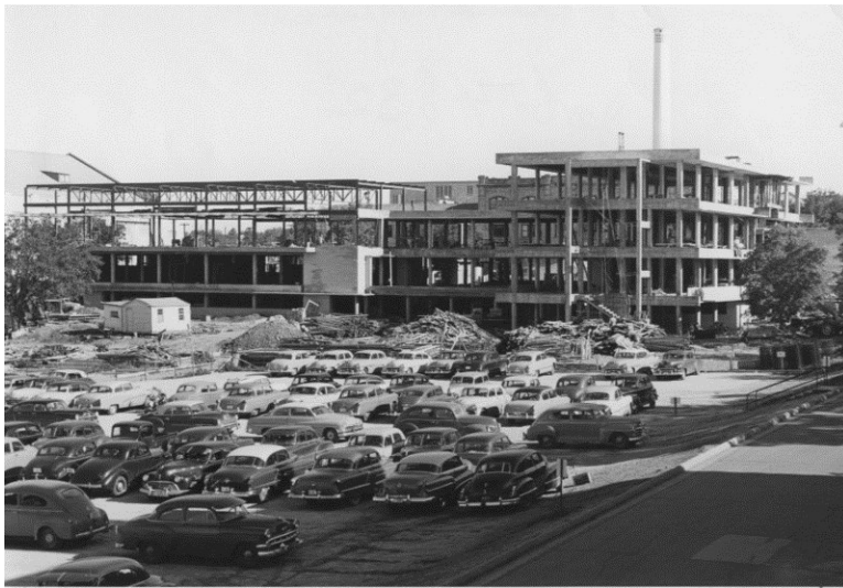
Union under construction
