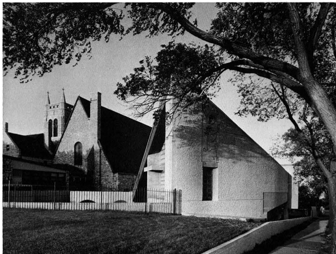
1. View of cathedral complex and sunken courtyard from freeway ramp.
