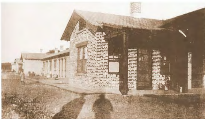
EL RANCHITO LADRILLO, SANTA FE RR EMPLOYEE HOUSING Florence Public Library
