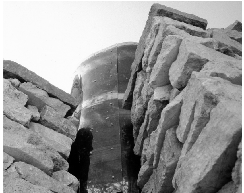
Detail of wall element
