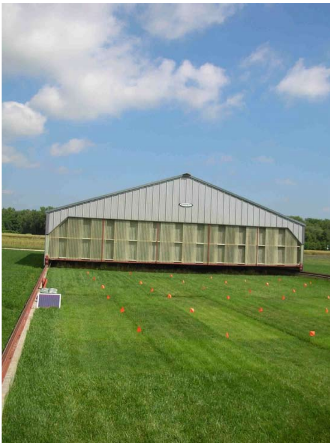
Figure 1. Rainout shelter (180 m 2 ) at Rocky Ford Turfgrass Research Center near Manhattan, KS. The rainout shelter automatically moved over plots (on tracks) when rainfall began, then retracted one hour after rainfall ended.
