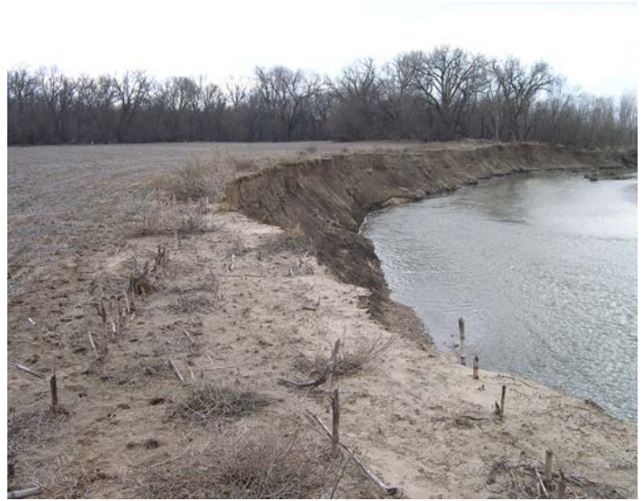
Figure 10 Streambanks lacking permanent vegetation are more susceptible to erosion.
